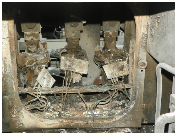
Fig.16 Cofret rele maxime de curent poz.54.1-3
