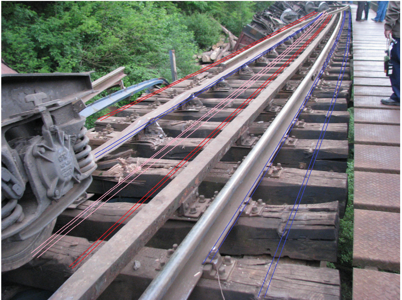
Photo no. 9 The traces left on the bridge by the derailed wagons
