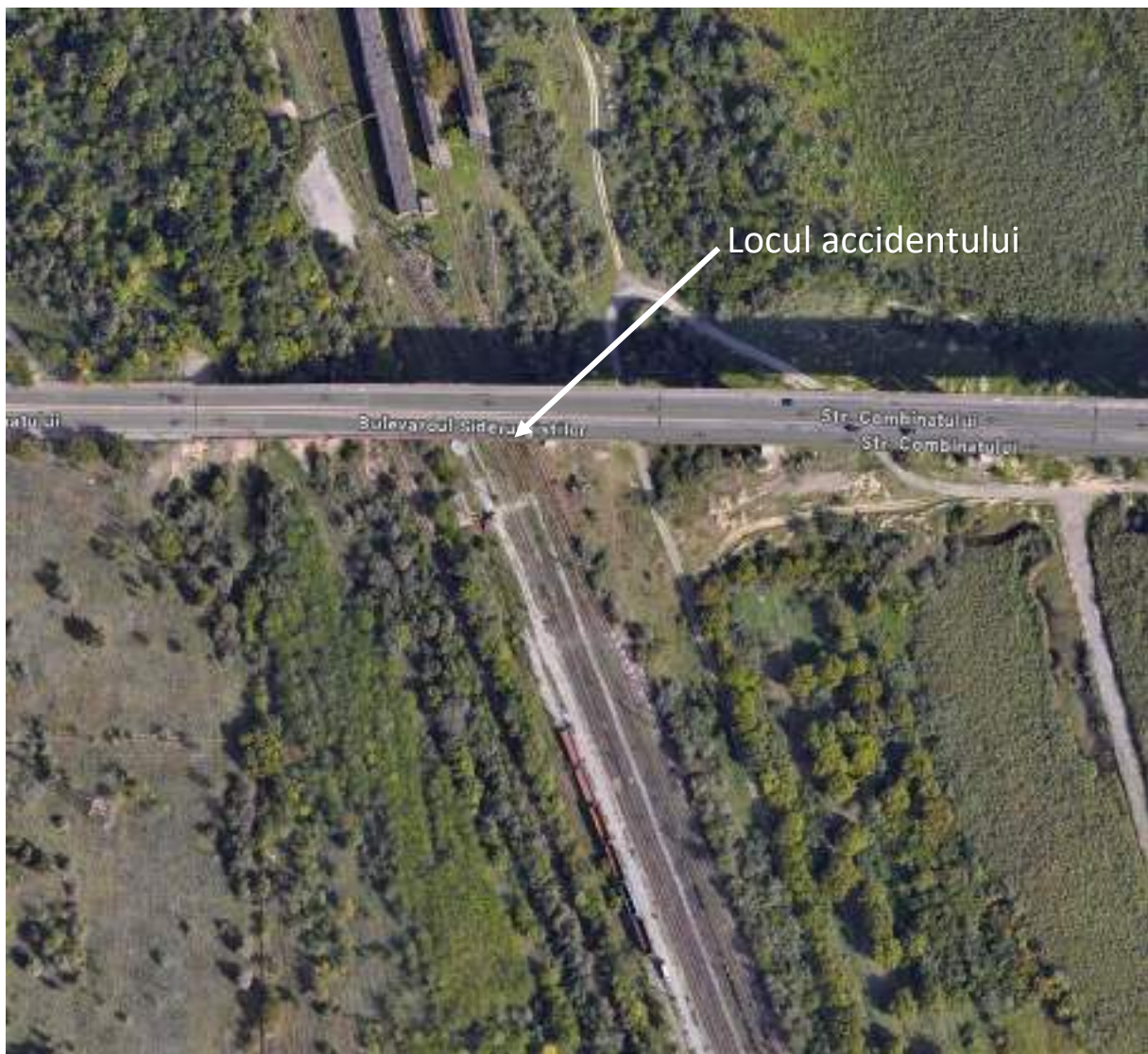
Figure no.1 Accident site
